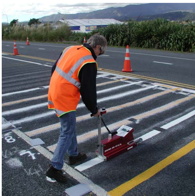
Measuring with the Zehntner instrument immediately after installation.
